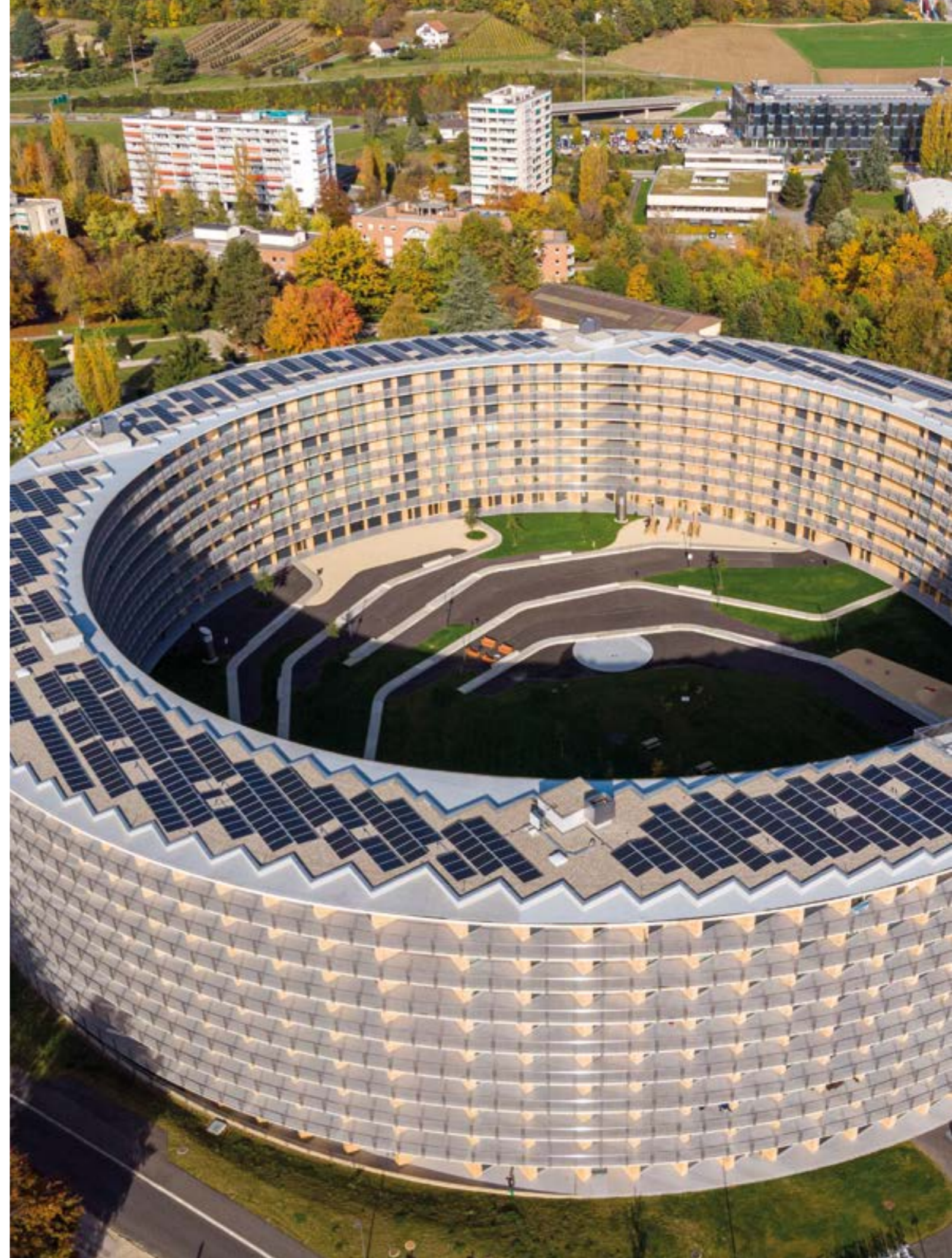
▲ Vortex Campus in Lausanne | High-performance modules with LOCKUP Flatport | 330 kWp | Image: Université de Lausanne
