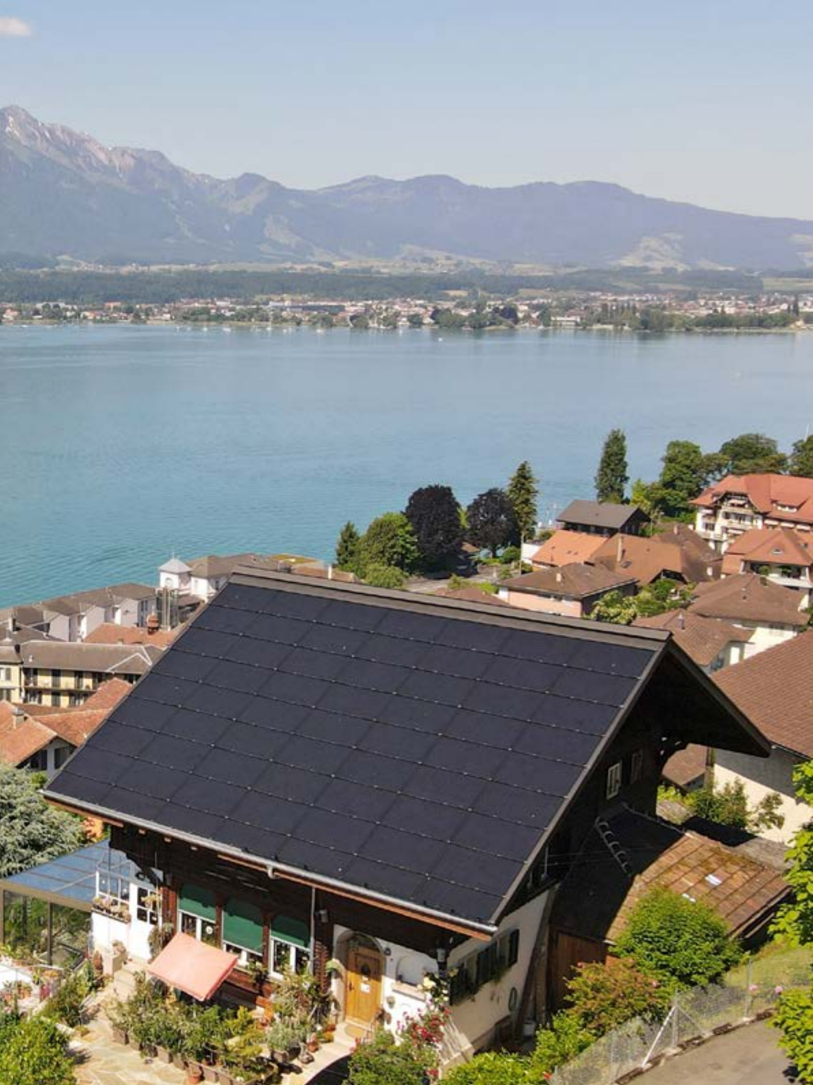
▲ Powerful chalet roof in Hilterfingen | LEVEL roof-integrated system
