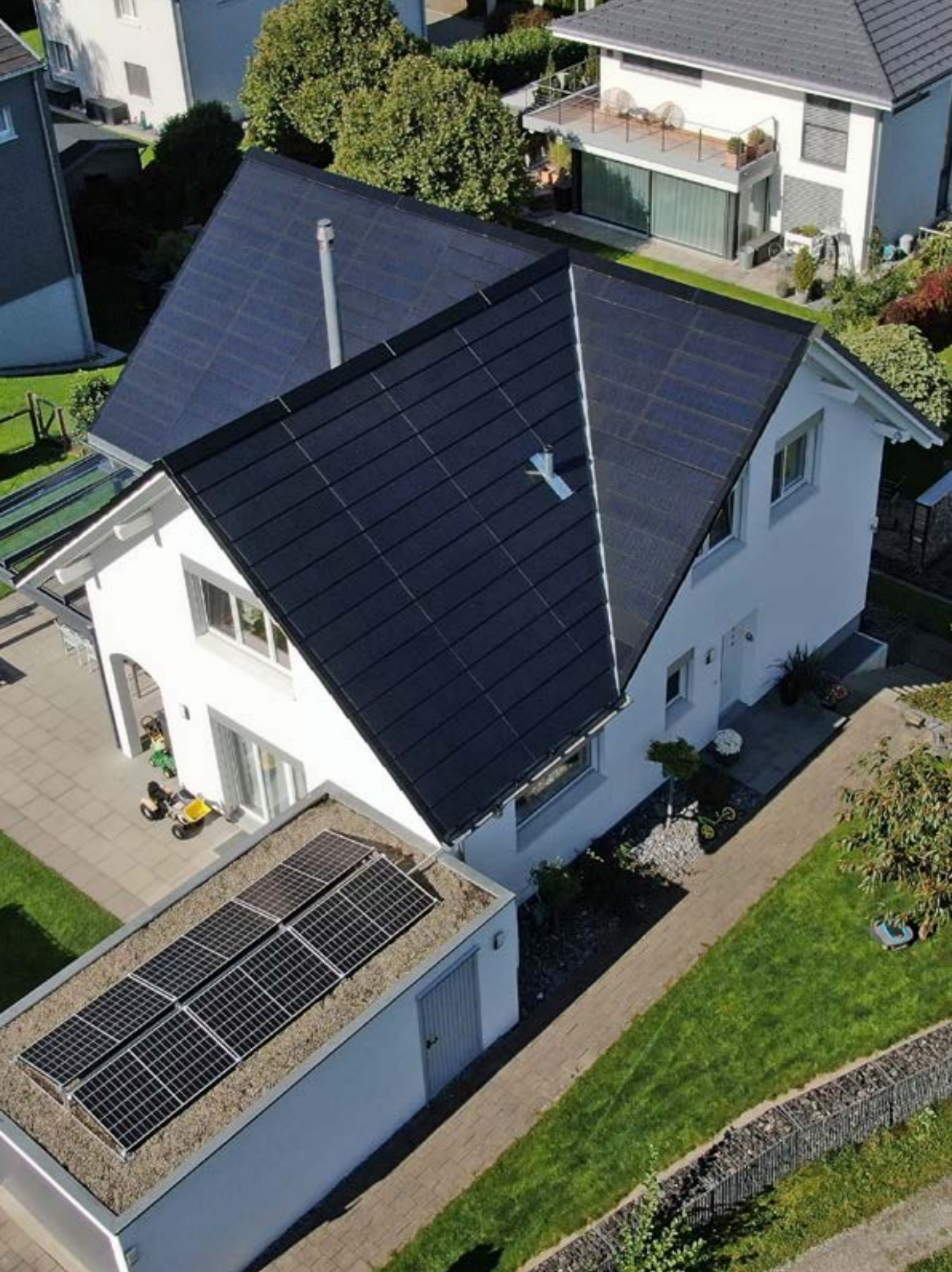
▲ Single-family house in Waldkirch | MATCH Slate roof-integrated system, next to it: a rooftop system on a garage.
