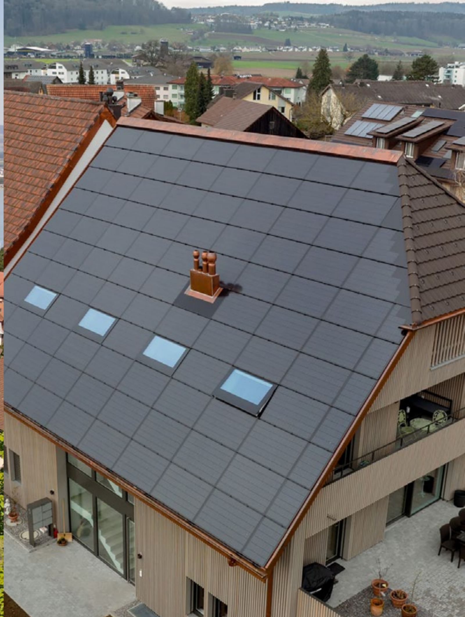
▲ Apartment building in Waltenschwil | LEVEL roof-integrated system
