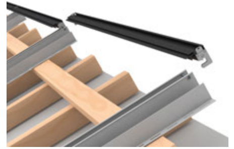
3 The ridge profiles are then installed.
