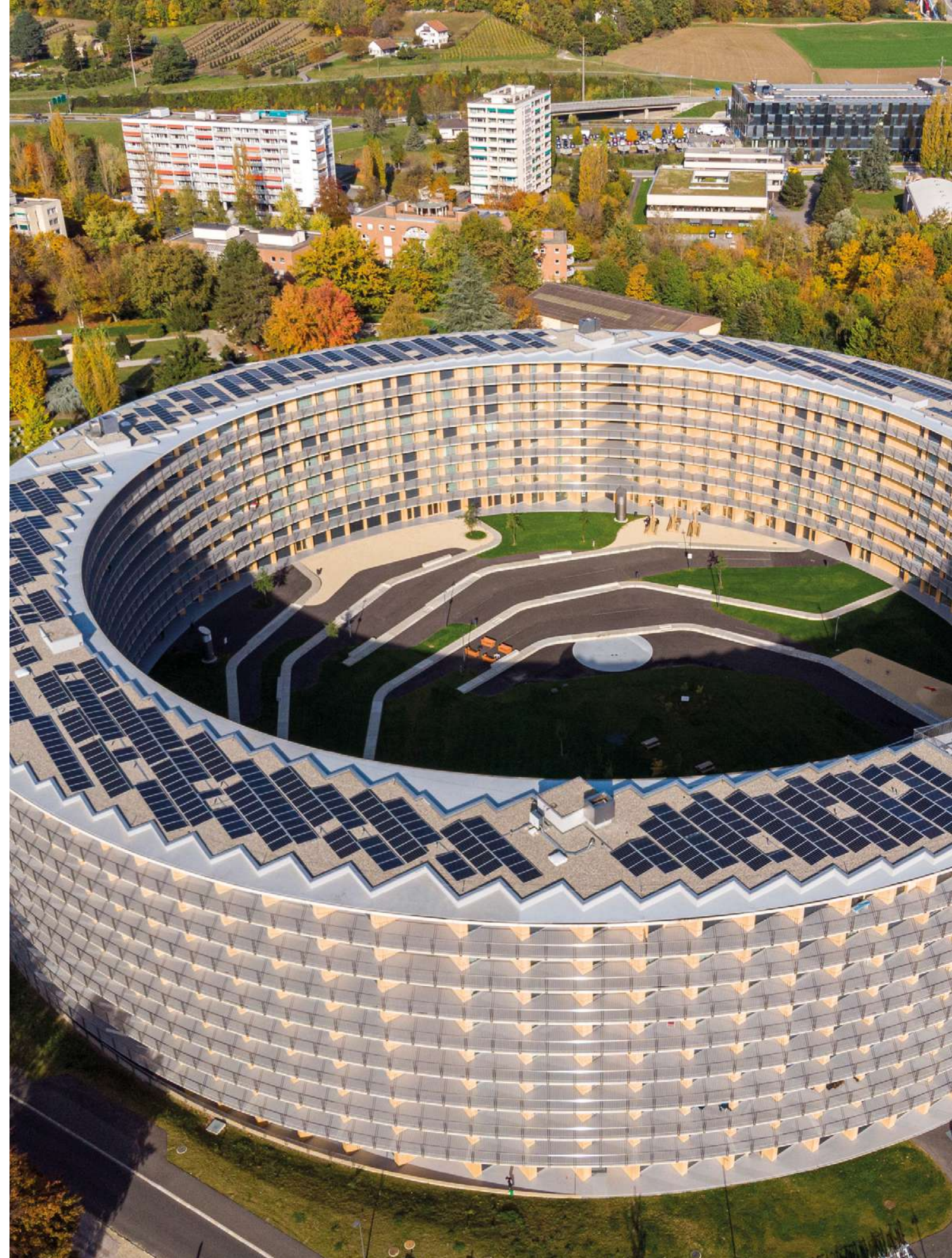
▲ Vortex Campus in Lausanne | High-performance modules with LOCKUP Flatport | 330 kWp | Image: Université de Lausanne
