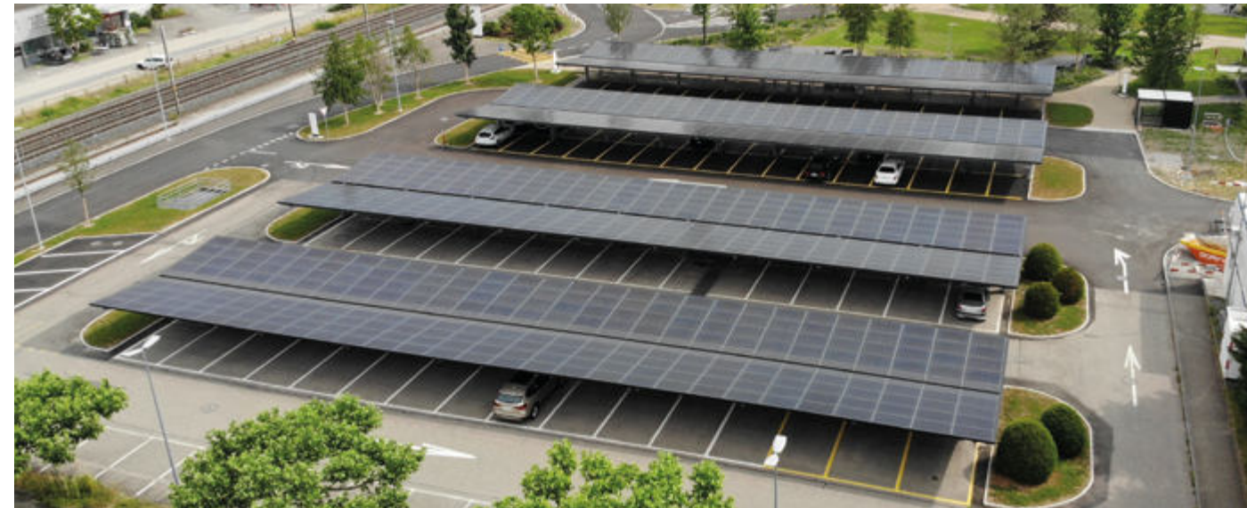
▲ Carport in Lucerne, CH | Plant capacity: 328 kWp
