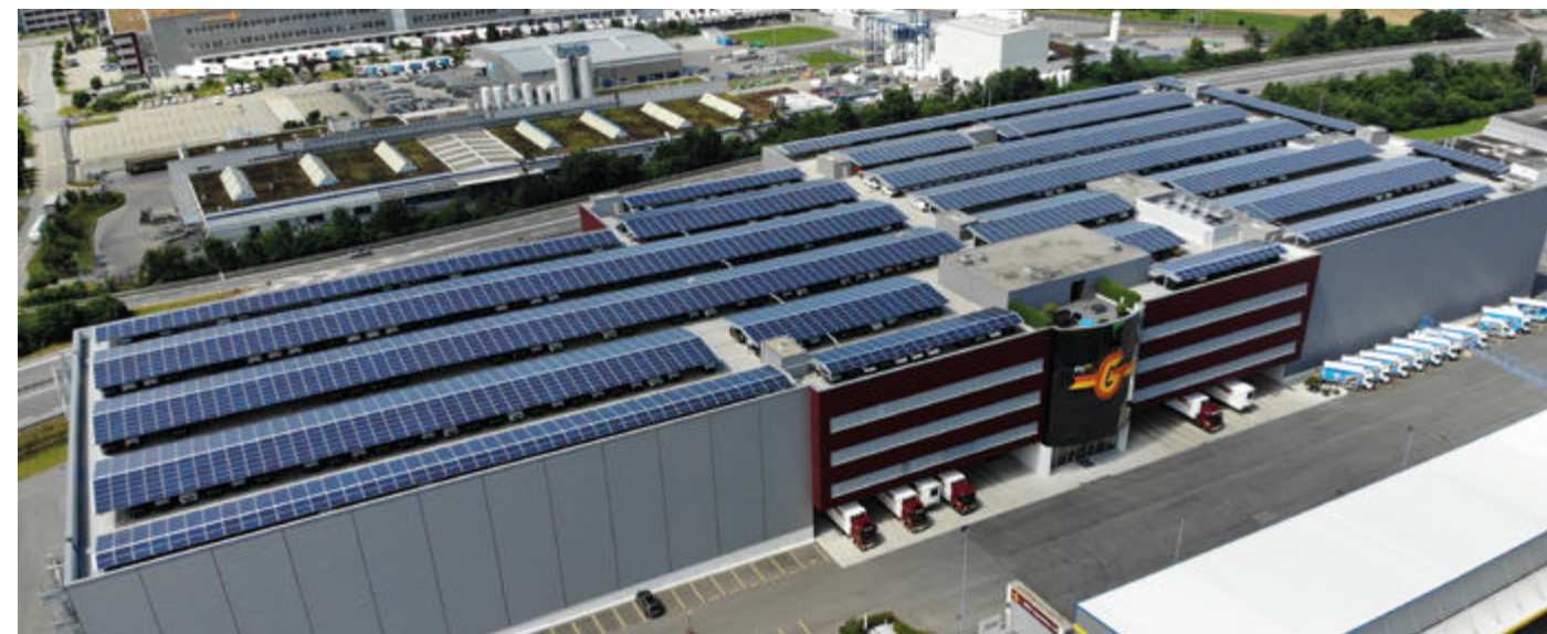
▲ Carport in Dagmersellen, CH | Plant capacity: 1.8 MWp
