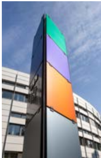
▲ BIPV demonstration stele Image: Fraunhofer ISE
