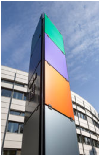
▲ BIPV demonstration stele Image: Fraunhofer ISE
