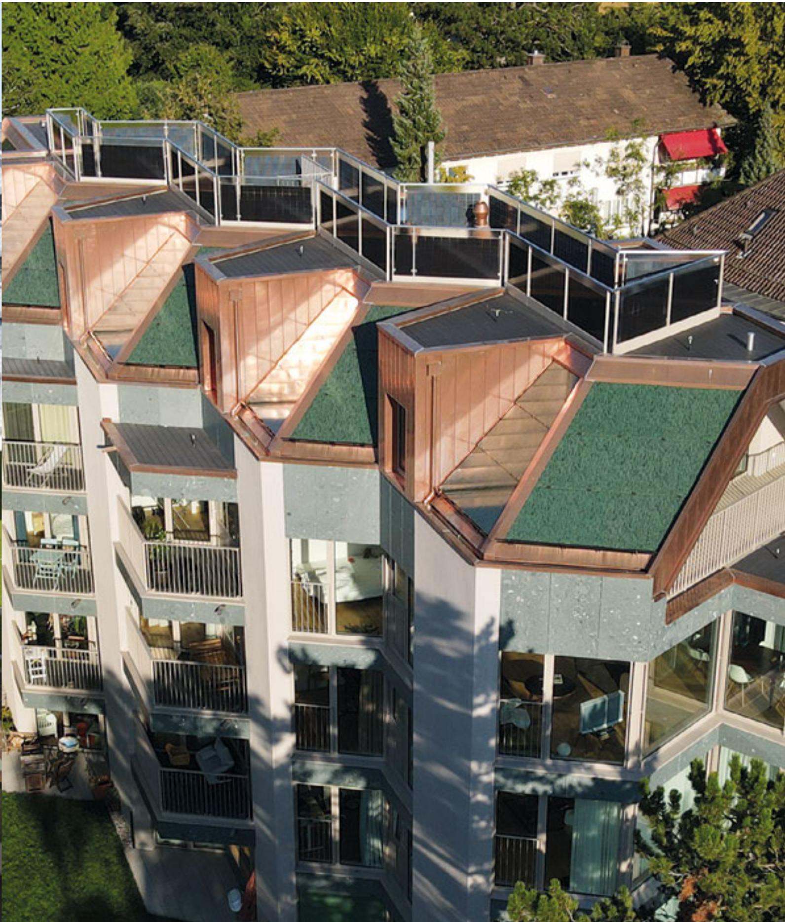
▲ Apartment building in Zurich | The LEVEL roof-integrated system anticipates the emerging patina of the copper roof in terms of color
