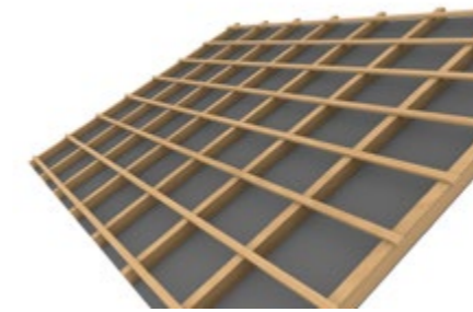
1 Prepare roof battening
