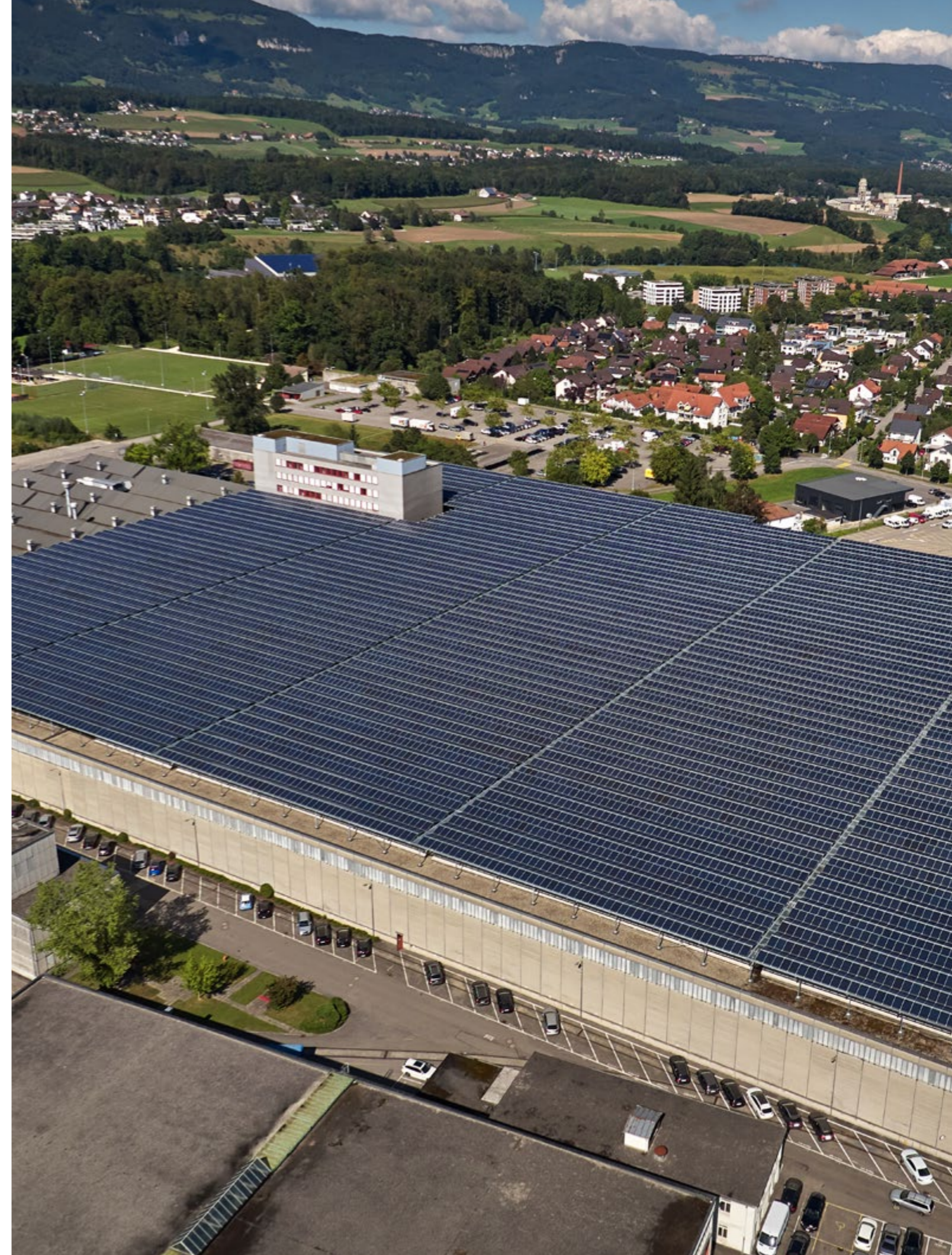
▲ Riverside Business Park Zuchwil | 36'000 m 2 | 5.76 MWp | Swiss Solar Prize 2016
