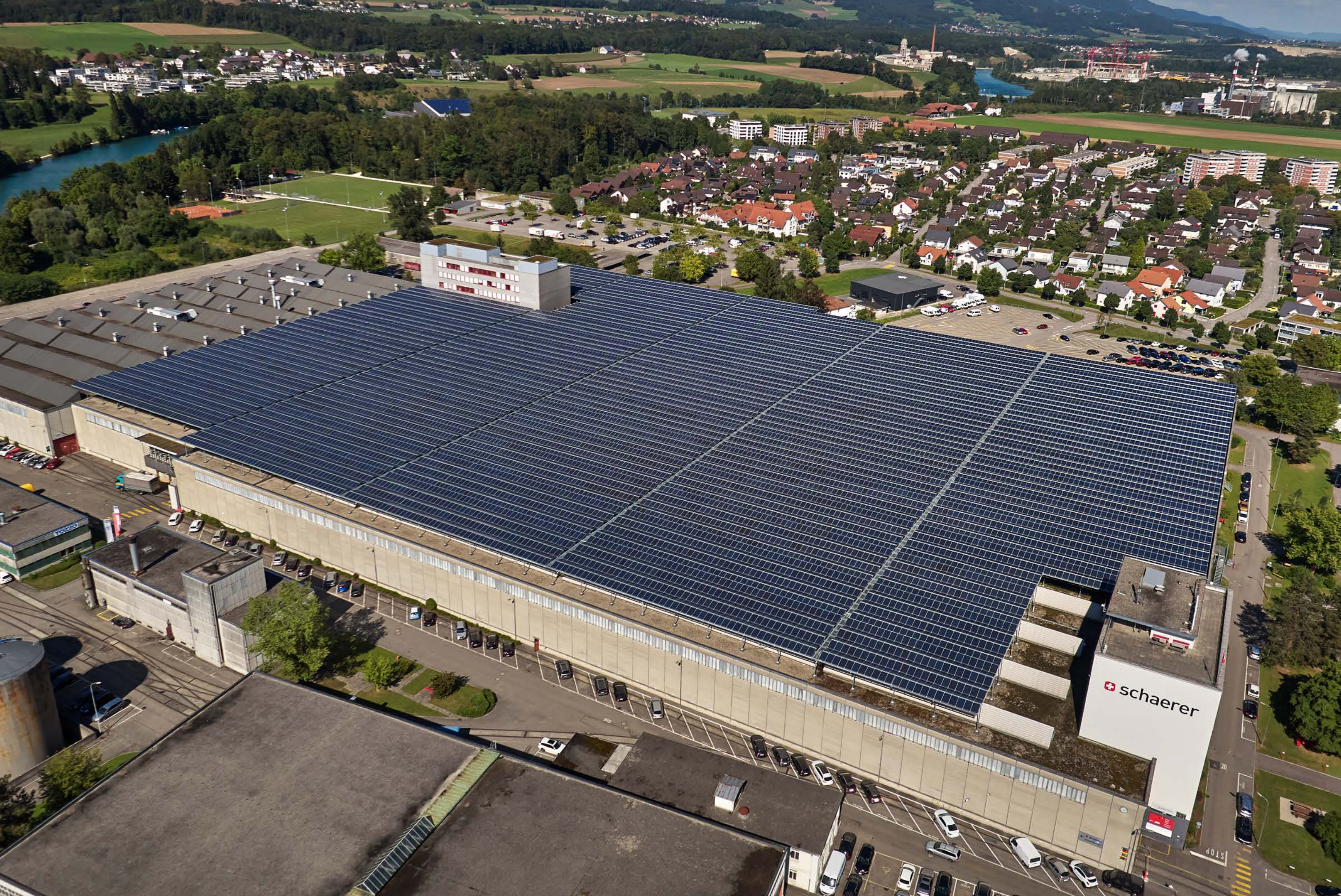
▲ Riverside Business Park Zuchwil | 36'000 m 2 | 5.76 MWp | Swiss Solar Prize 2016
