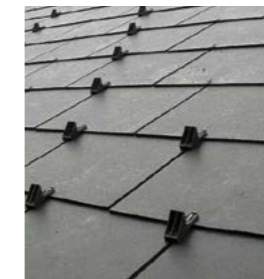
Fibre cement roof
